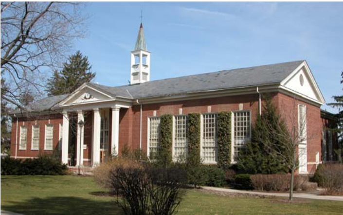
The Blough-Weis Library in 2008, entrance facing West.
